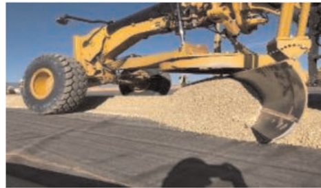
Figure 4b. Equipment and material over BGM.
