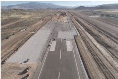
Figure 4a. General view of the site.
