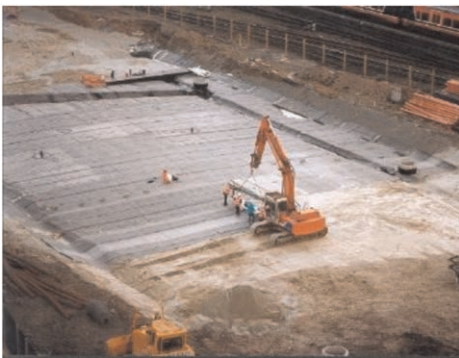
Figure 8a. Membrane installation.
