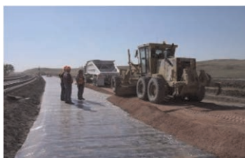
Figure 6b. Sub ballast placement directly on BGM.
