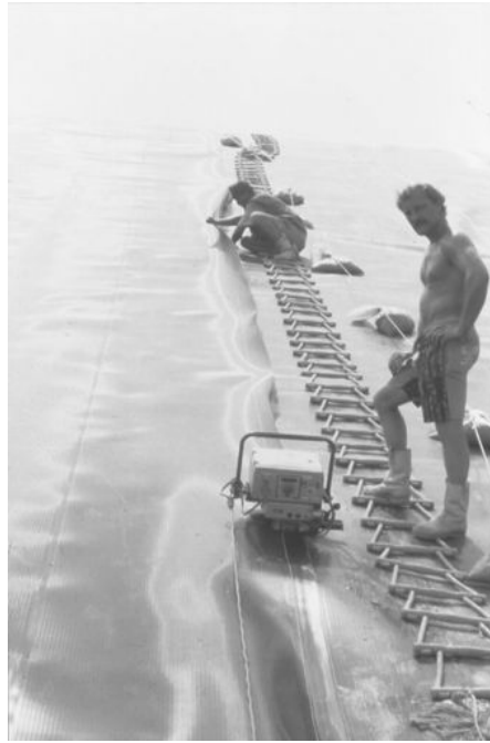
Figure 17.14 Photograph of a wedge welder seaming HDPE geomembranes on a steep slope. Reproduced by permission of NAUE
