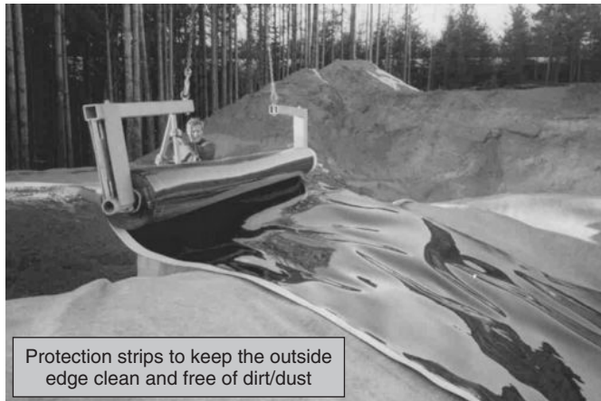
Figure 17.29 Photograph of a specialty HDPE geomembrane showing the white protection strips on the edge of the geomembrane to keep the edge clean and free of dirt/dust for welding. Reproduced by permission of NAUE
