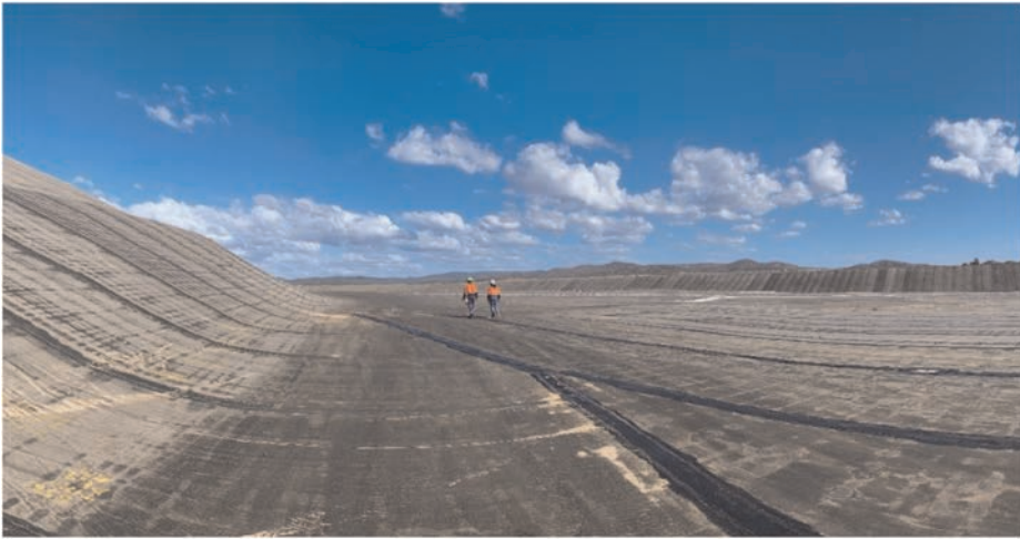
Figure 8. Ravenswood Gold tailings storage facility.
