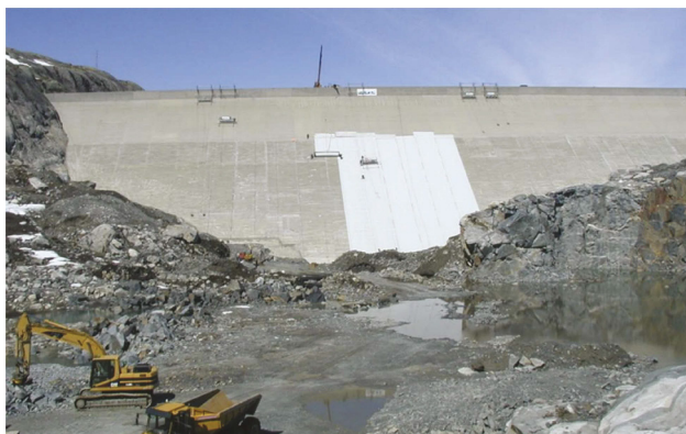
Figure 8. Rehabilitation of Midtbotnvatn rockfill dam in Norway: placing of PVC composite geomembrane layer over the damaged cement concrete facing.
