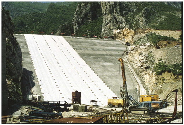
Figure 6. Bovilla dam: composite geomembrane placing over the porous cement concrete layer.
