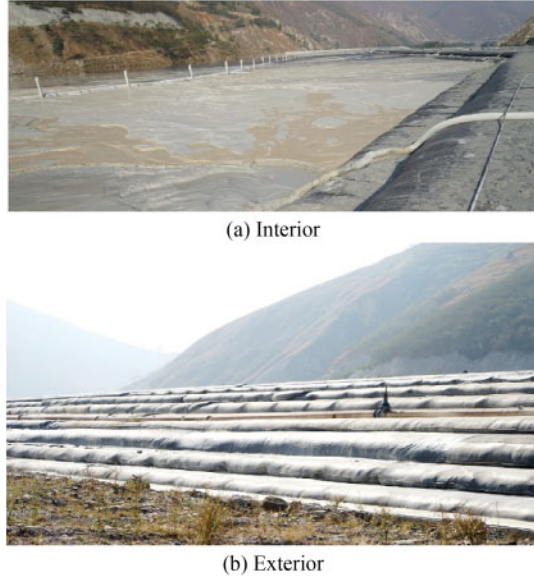
Figure 1. Zoomed-in partial view of tailings dam: a) interior; (b) exterior.
