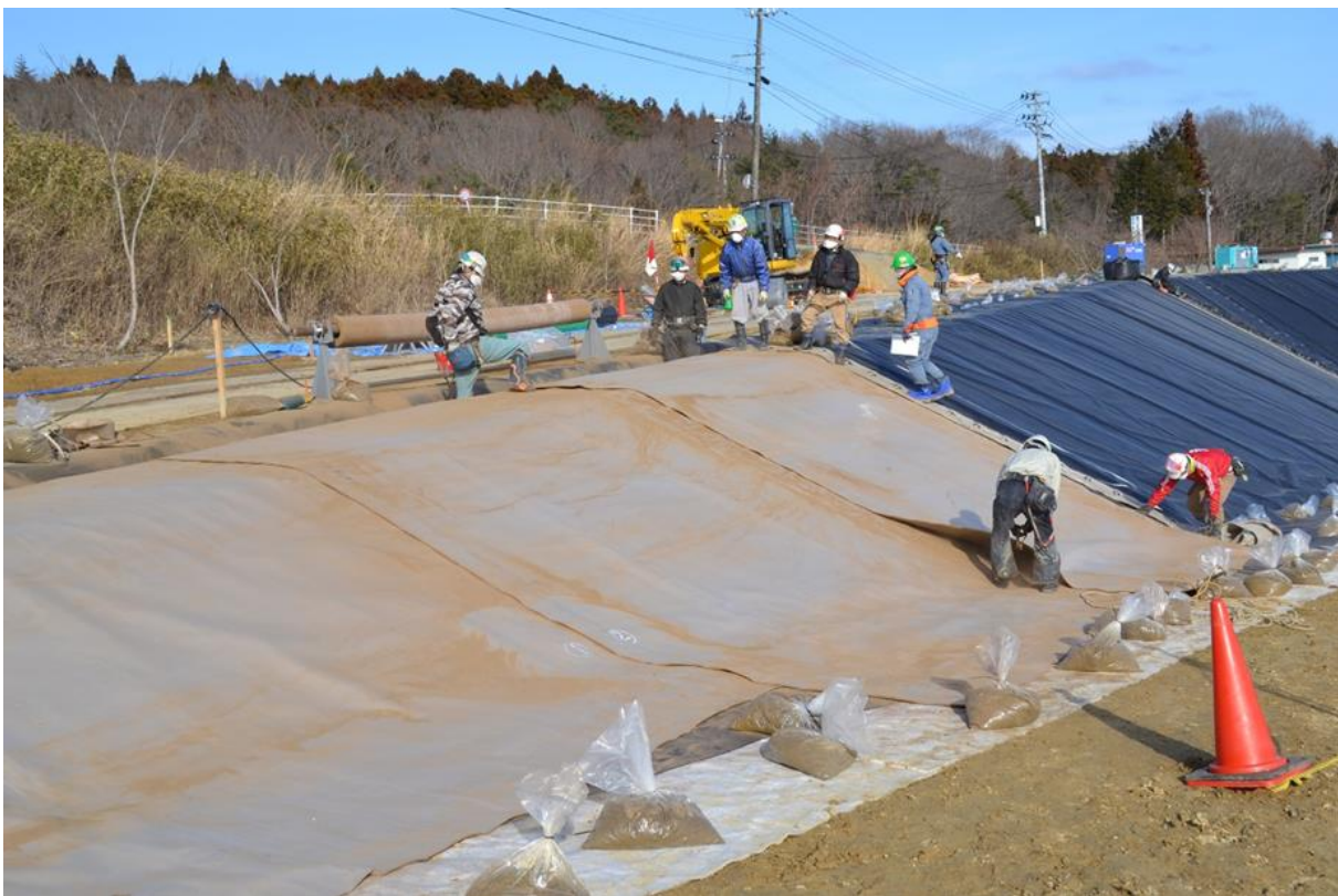
Fig. 8 Installation of the PE extrusion-coated multicomponent geosynthetic clay liner
