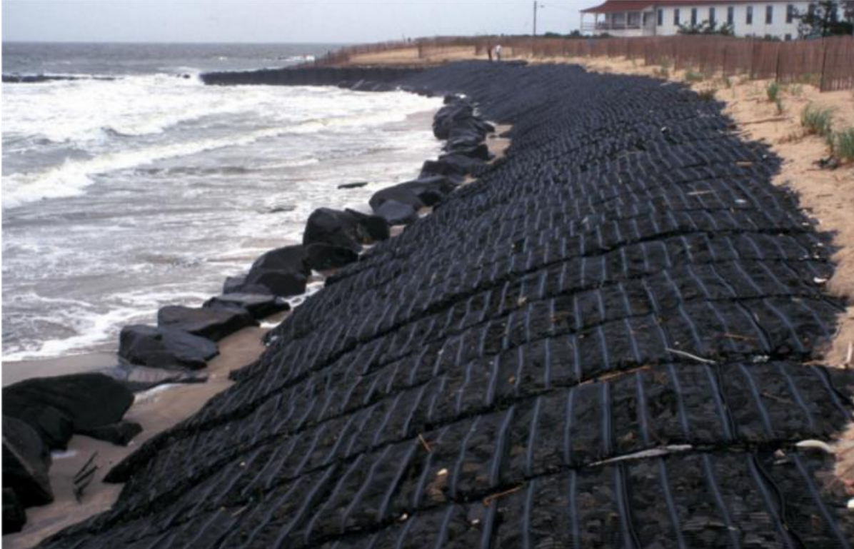
Figure 1. Typical Marine Mattress installed along a shoreline (Source: Hughes 2006).
