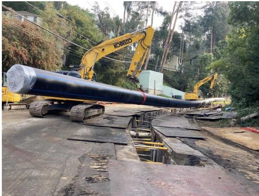
Figure 6. Walking the 36-inch HDPE Pipeline into Position
