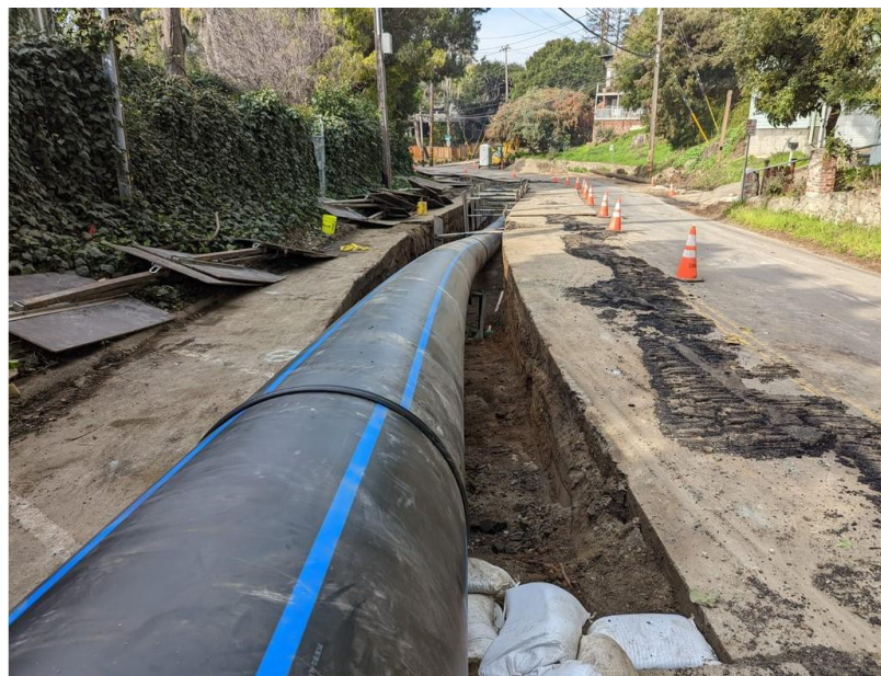
Figure 7. Pushing the 36-inch Pipeline into the Trench
