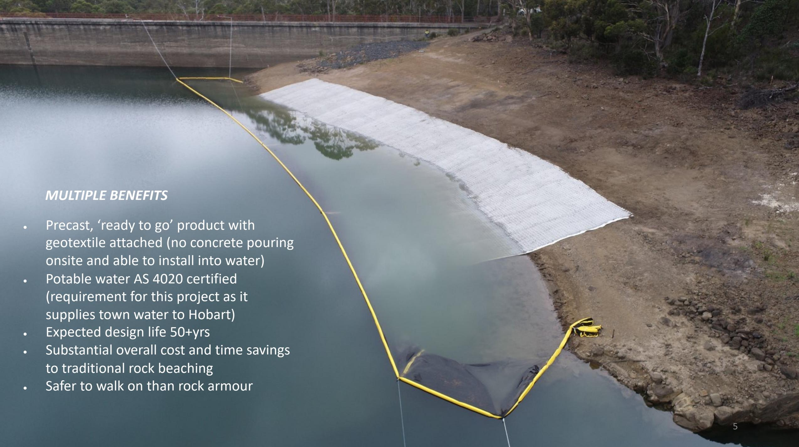
An aerial photograph showing a dam structure on the left. A large, rectangular, white geotextile mat is being installed in the water, extending from the dam towards the right. The mat is held in place by a yellow floating barrier. The water is calm, reflecting the sky and the surrounding trees. The right bank is a mix of dirt and rocks, with some vegetation. The overall scene is a construction site for a water treatment or containment structure.
