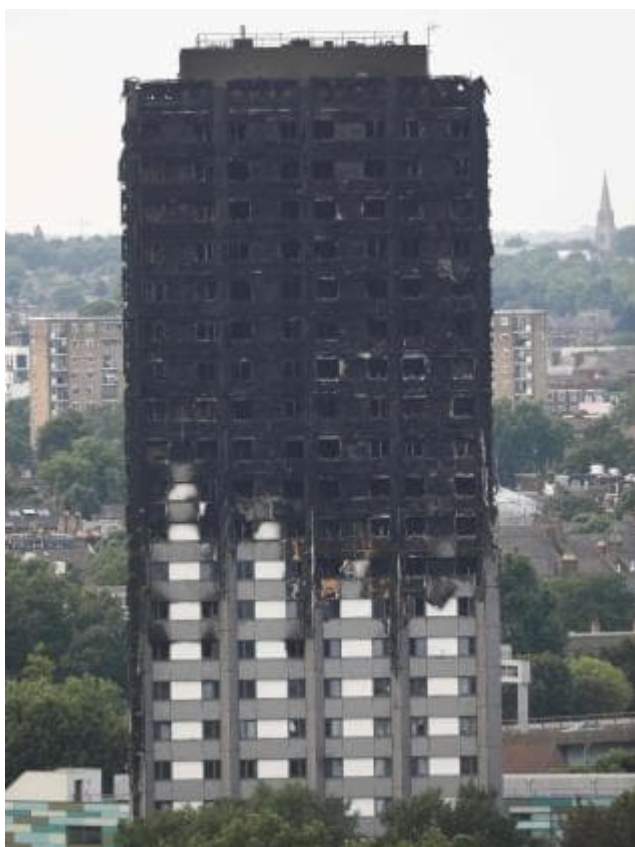
Figure 3 (FILES) In this photo taken on June 18, 2017, unburned lower floors with untouched cladding in place are seen with the burnt out upper floors of the Grenfell Tower block in North Kensington, west London. / AFP PHOTO / Tolga AKMEN
