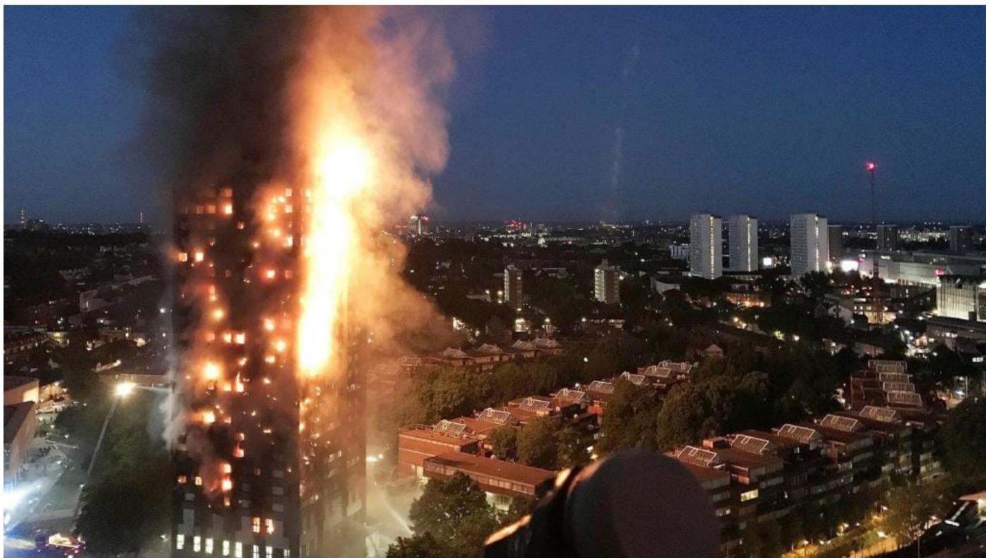
Figure 2 In this image taken by eyewitness Gurbuz Binici, a huge fire engulfs the 24 story Grenfell Tower in Latimer Road, West London on June 14, 2017.
