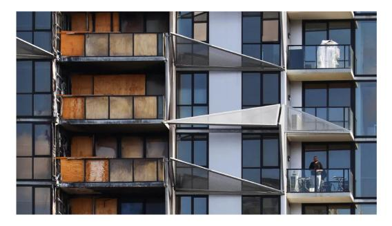
The Lacross building in Docklands, where flammable cladding was used, suffered serious damage in an out-of-control fire. Picture: Aaron Francis
