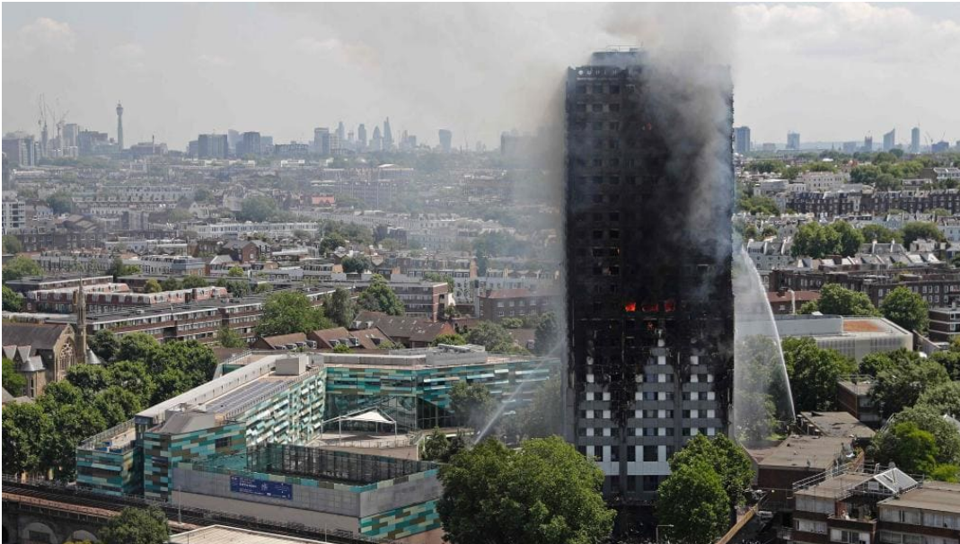
Figure 2 ABC bosses investigated the cladding after Grenfell Tower blaze in London. / AFP PHOTO / Adrian DENNIS
