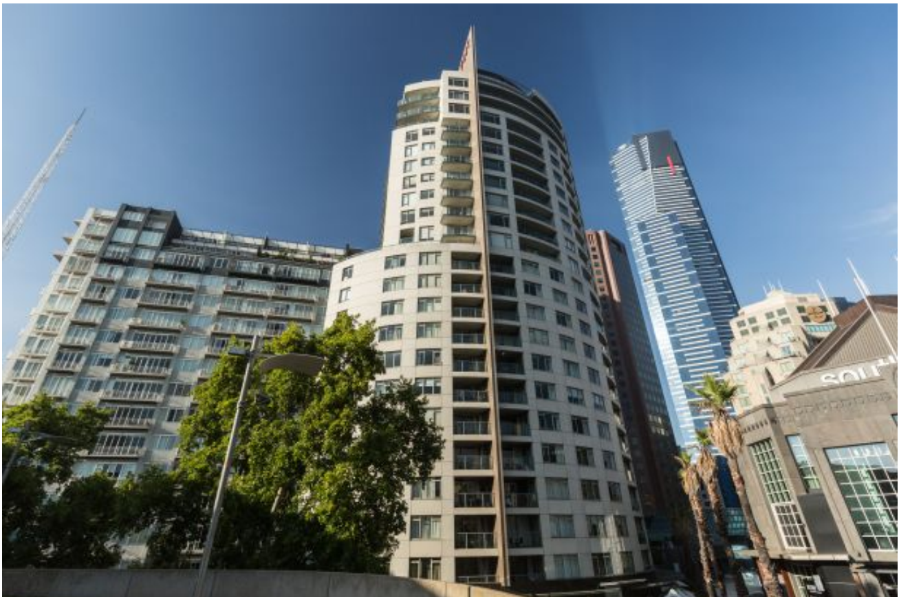
The Quay West tower in Southbank, Melbourne. It has a fin made of flammable cladding that Melbourne
