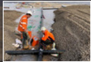
LEACHATE PIPE WORK
