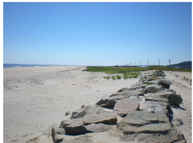
Fig. 3 Accretion of beach and dune at Sandy Hook, New Jersey following a large scale beach nourishment project. The seawall was initially built in the early twentieth century (Dallas et al. 2013). Accretion over the seawall in the distance was aided by a landward recurve in the seawall that provided a wide beach that facilitated aeolian transport
