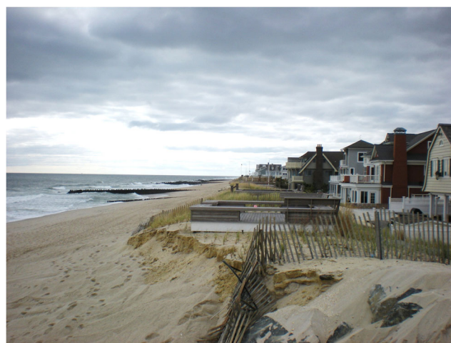
Fig. 6 Buried seawall at Bay Head, New Jersey October 2015, showing condition 3 years after the sediment cover was removed during Hurricane Sandy in October 2012. The height and location of the seawall is revealed in the exposed segment at the municipally-maintained portion in the foreground
