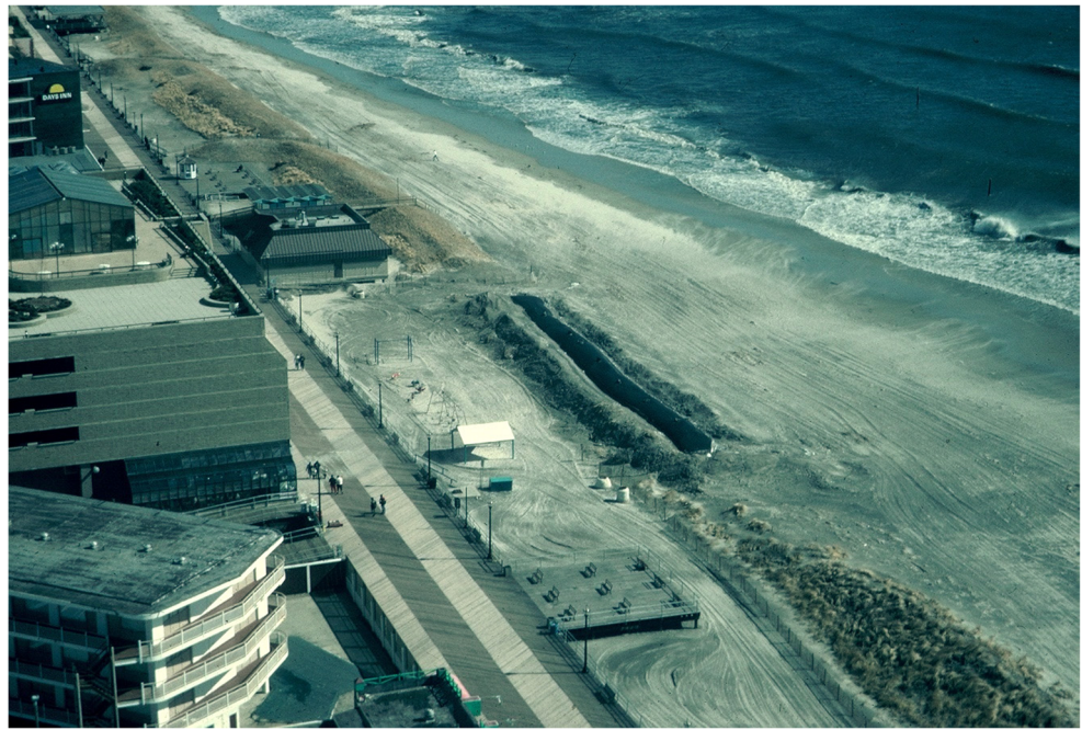
Fig. 1 Geotube being repaired at Atlantic City, New Jersey in March 1996. The dunes to either side of the installation site are similar geotubes covered by bulldozed sand
