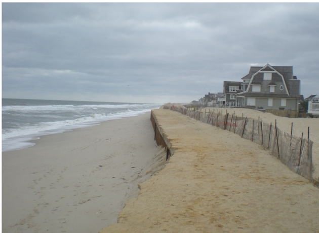
Fig. 2 The exposed portion of the 5.6 km-long steel bulkhead built at Mantoloking, New Jersey in October 2016. The bulkhead was built after erosion caused by Hurricane Sandy in October 2012. The sand cover initially placed over the structure has eroded. Fence placement well landward of the structure reduces the risk of accidental fall. A beach nourishment operation conducted in the winter of 2017–2018 subsequently restored the beach and allowed aeolian accretion to occur
