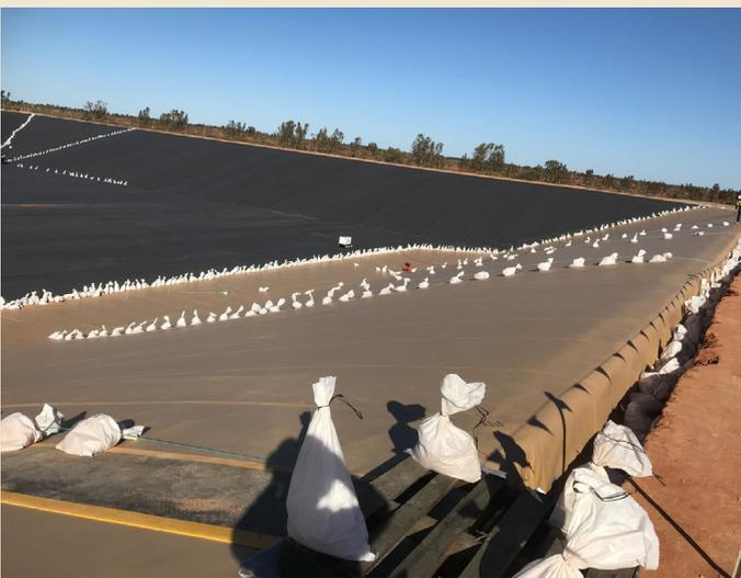
CSPE primary liner (brown) being installed over the conductive geotextile
