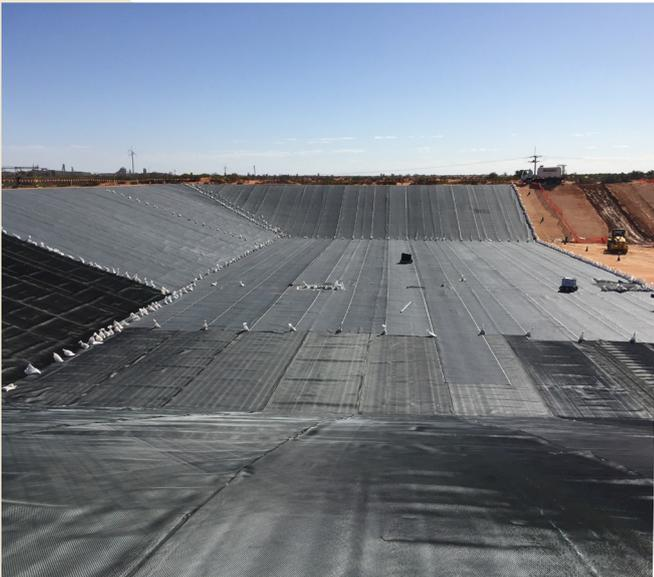
Geocomposite drain and conductive geotextile being installed
