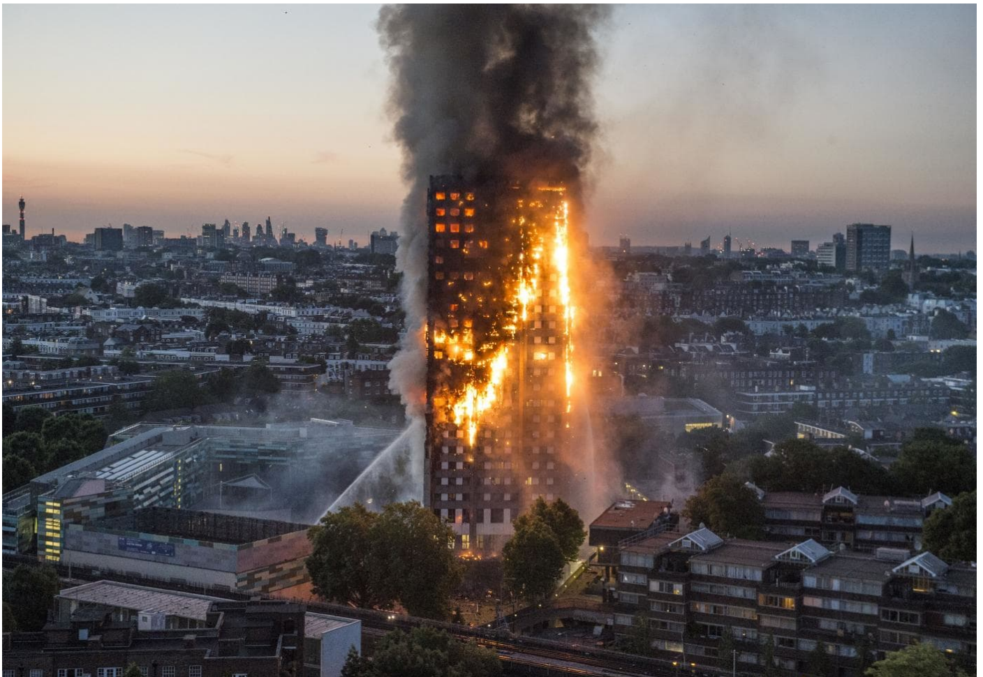
Figure 1 The Grenfell Tower inferno sparked widespread calls for a cladding fire safety audit. Picture: Jeremy Selwyn/Evening Standard
