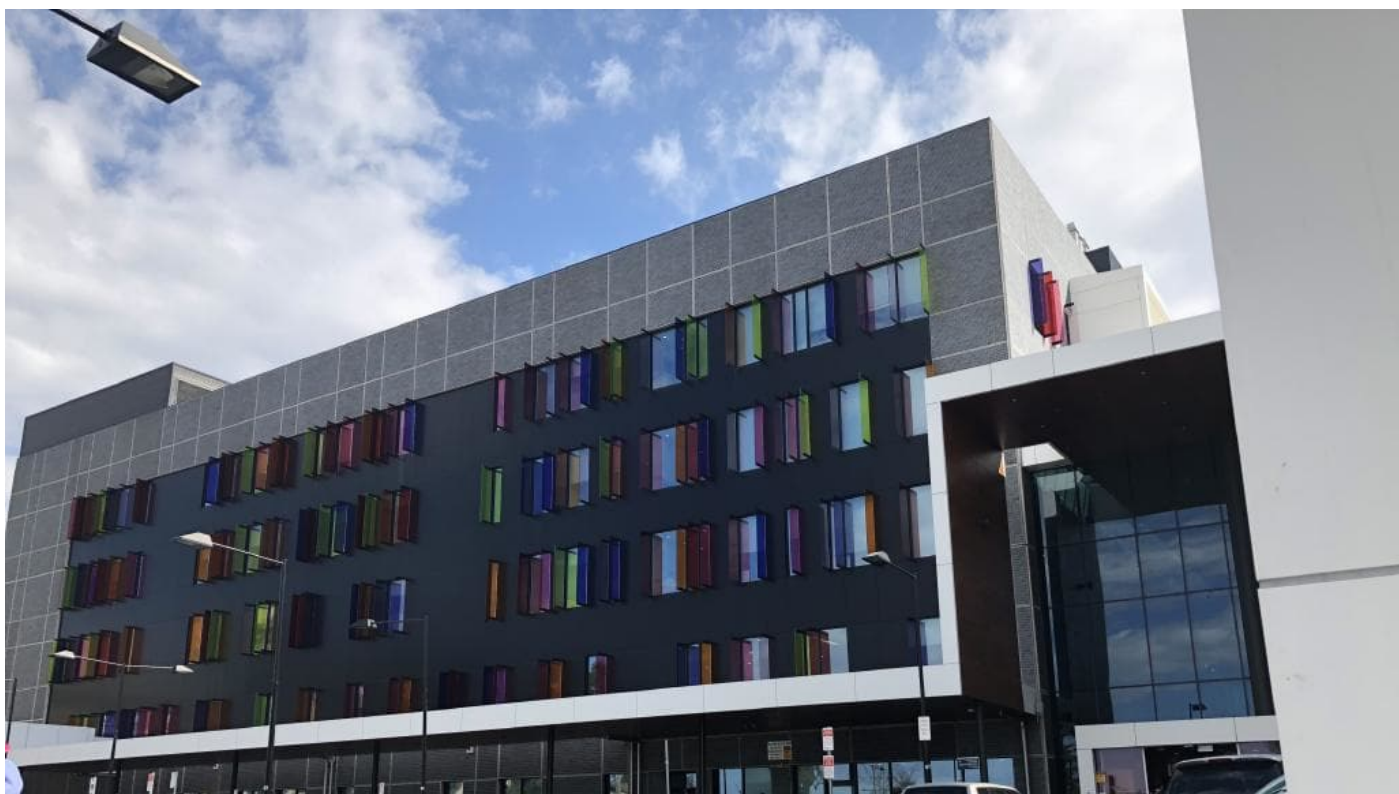
Figure 4 Cladding at Blacktown Hospital has come under scrutiny.
