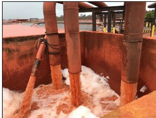
Figure 4.12 Effluent box in DRS1 showing permanent and mobile pumping into the box
