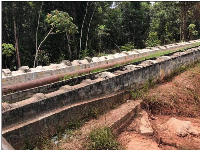
*Figure 4.14 Effluent pipes in Area 45, steel pipe from DRS2 shown in the middle*
