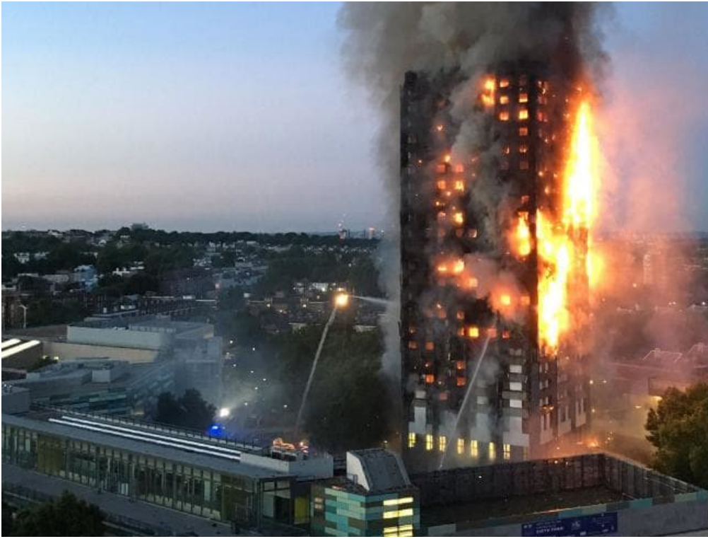
Figure 2 The blaze at Grenfell Tower last year. Picture: Natalie Oxford
