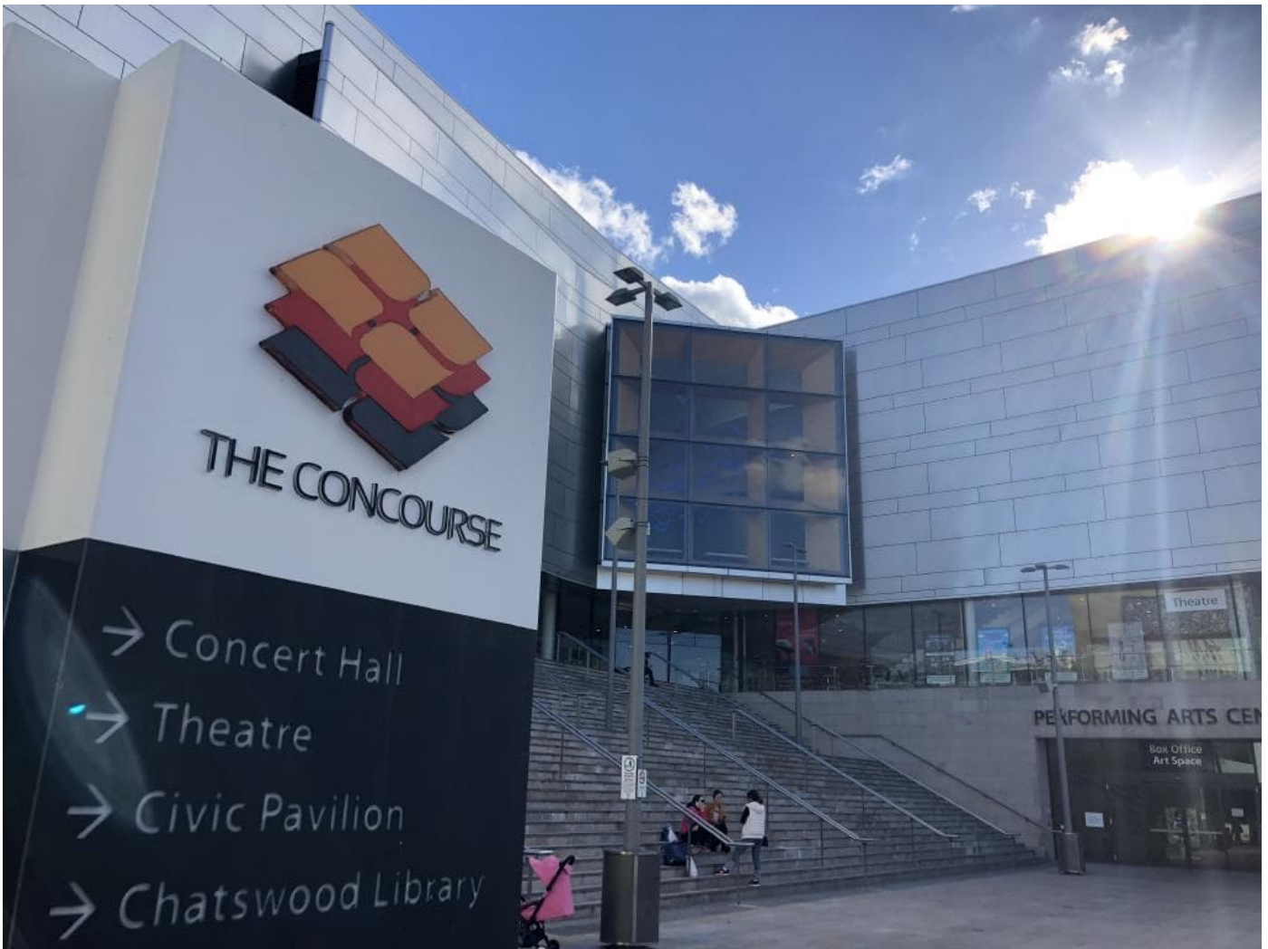
Figure 1 The Concourse at Chatswood is cladded is similar to that which contributed to a London tower fire last year in which 72 people died.
