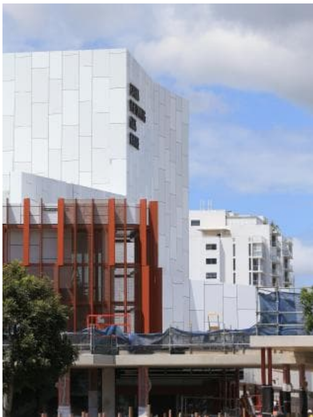
Figure 1 QFES has raised grave concerns about the use of potentially flammable insulation and cladding in the Cairns Performing Arts Centre. PICTURE: JUSTIN BRIERTY
