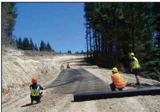
Figure 5. Placing a 25-m long section of geogrid into position.
