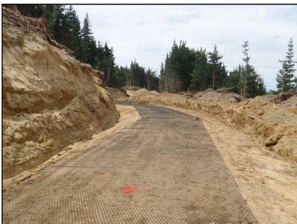
Figure 6. Geogrid placement to fit a curve on a forest road.
