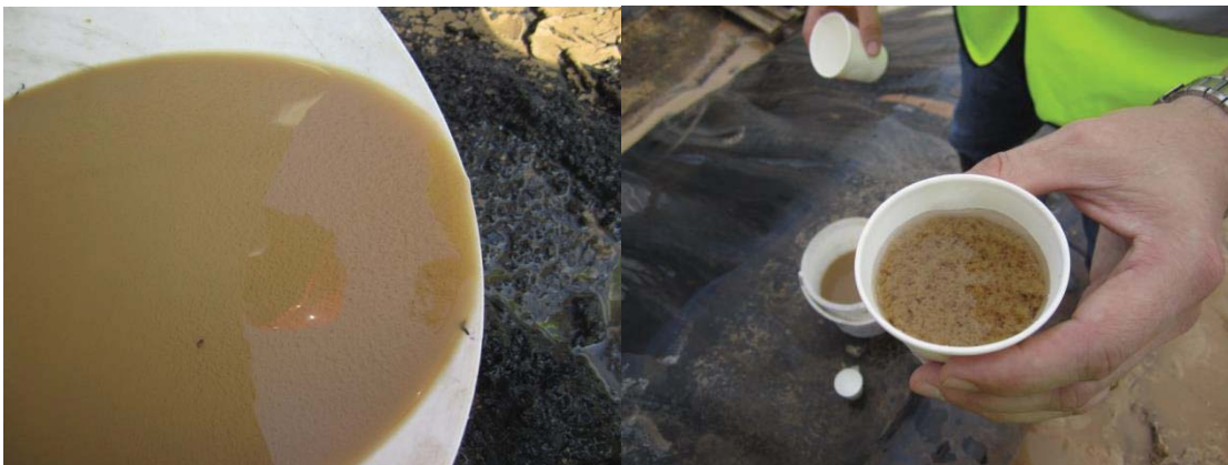
Figure 5. Influence of polymer admixture: Not properly treated slurry (left hand side); Proper flocculated sludge (right hand side).
