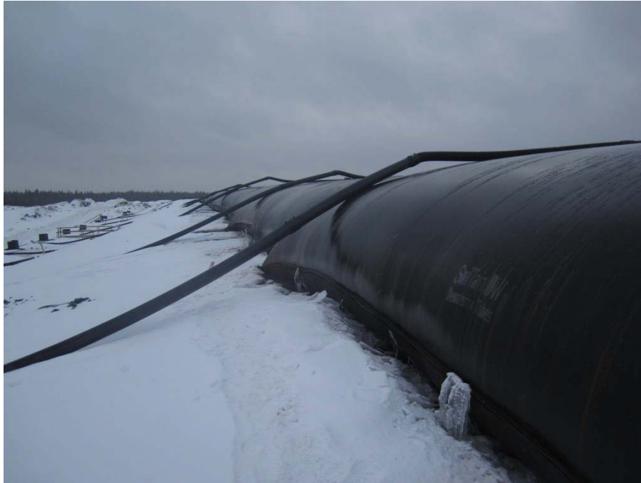
Figure 6. Operation of the additional placed fifth tube layer during winter; the four tube layers below are completely covered by snow and ice.
