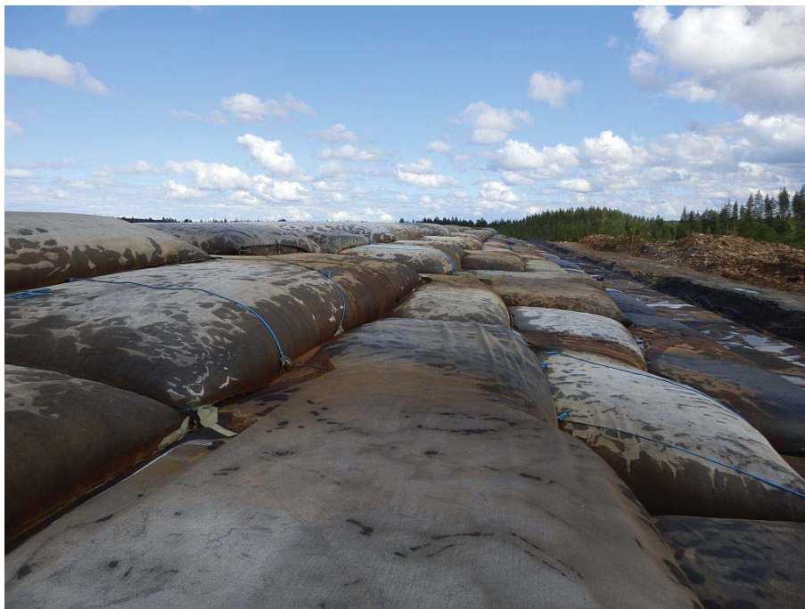
Figure 7. Completed dewatering field with fifth tube layer.
