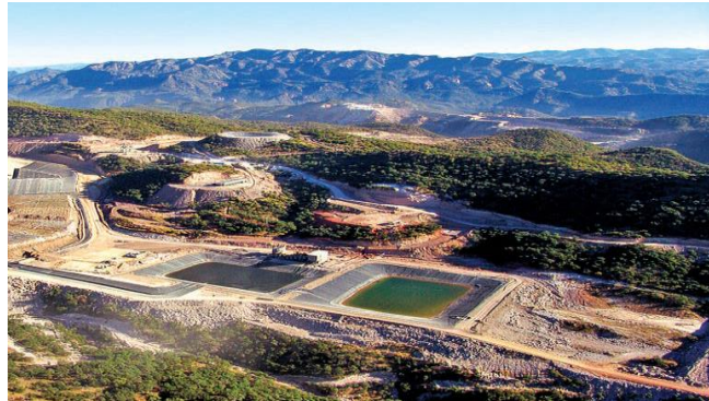
Fig. 2. GCL Placement in a Heap Leach Pad (Geosynthetic Materials Association, 2010)
