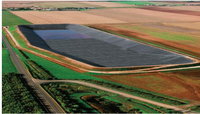
Fig. 5. GCL Placement in a Surface Impoundment (Geosynthetic Materials Association, 2010)
