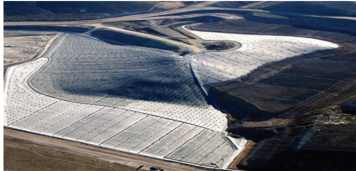
Fig. 3. GCL Placement as a Landfill Cap in a Closure System (Geosynthetic Materials Association, 2010)
