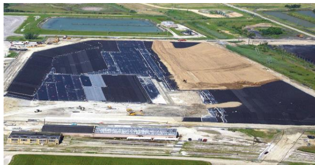
Fig. 1. GCL Placement in a Solid Waste Landfill (Geosynthetic Materials Association, 2010)
