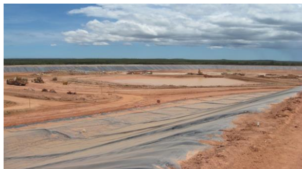
Fig. 9. GCL Placement in a Mine Tailing Dam (GDT Lining, 2017)
