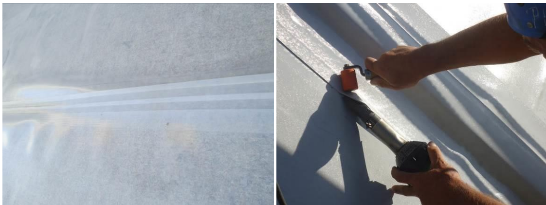
Figure 5 – Implementation of P-PVC welding: double weld, manual weld
