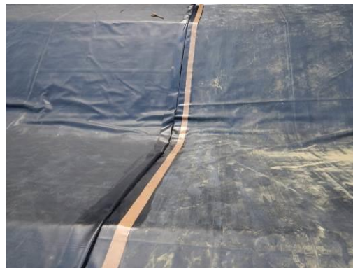
Figure 8 – Welding with EPDM
