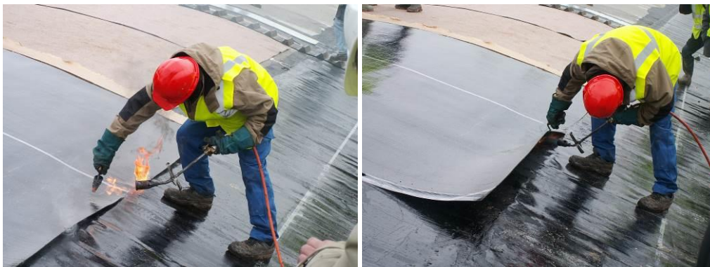
Figure 7 – Welding of bituminous geomembranes
