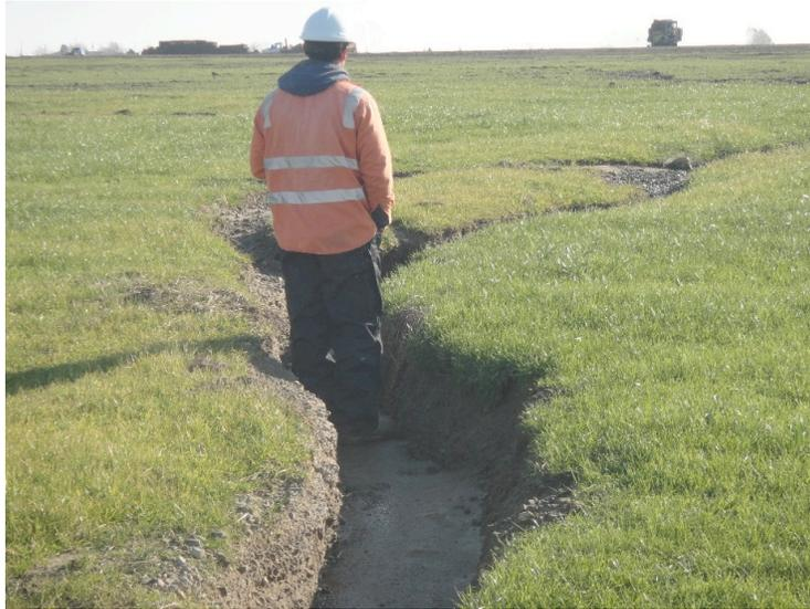
Figure 12. Seepage erosion feature on the Summit cover system exposing geotextile protector fabric and above geomembrane layer.
