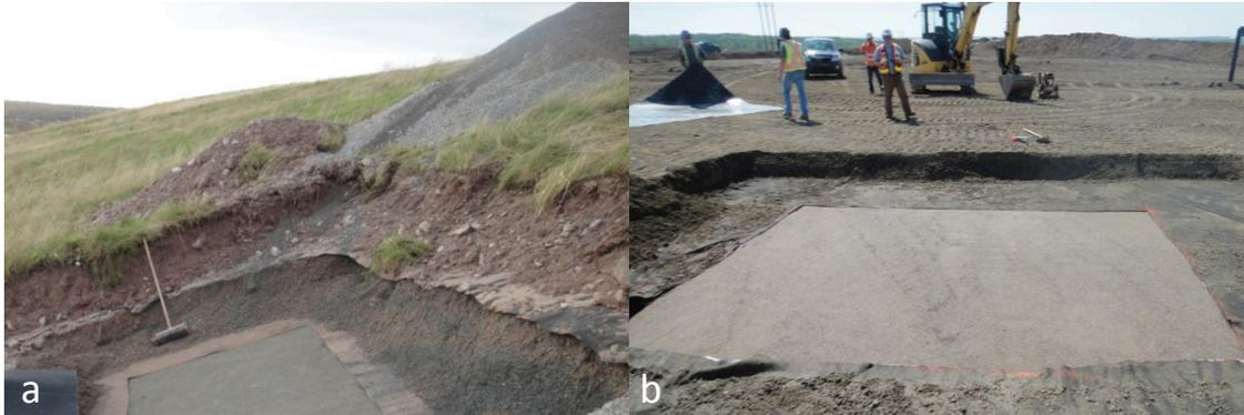
Figure 6. Exposed bedding sand at VJ (a) and Summit (b).
