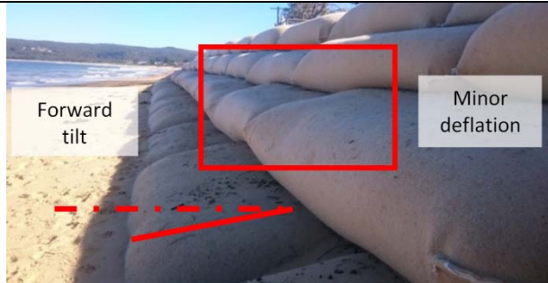
Figure 5: Evidence of minor deflation and “forward tilting” of geocontainers (photo taken 29 th June 2016)
