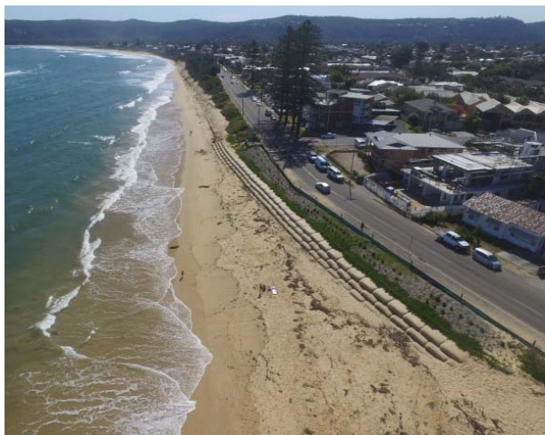
Figure 8: Photo of the CSG seawall looking west after one year in operation (Photo date:25/10/2016).
