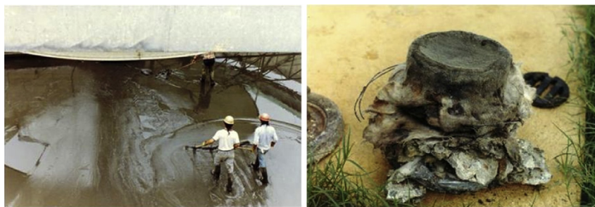
Fig. 6. Oily wastewater sludge clogging geotextile covered drains (GSI photos).
